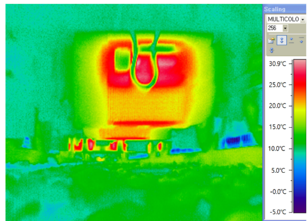
(b) IR thermal image for non-cooling IR camera
