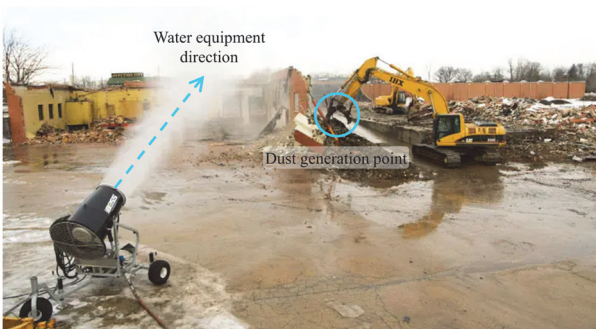
(b) Water spraying equipment shuttling in a demolition site
